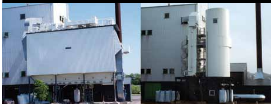
Figure 1: space optimisation – before (left) and after (right)
