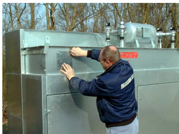
Fig. 3. Before re-securing the cover, make sure that the sealing is intact. If not, it should be replaced.
