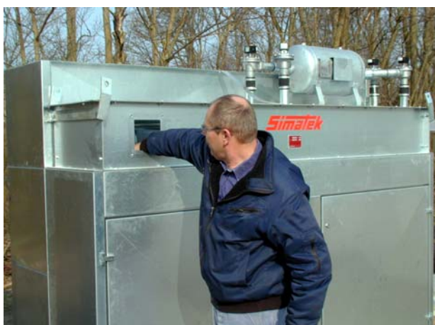
Fig. 2. The inspection hole is used when installing the last bag/cage and when removing the first cage. The bag installation should be planned so that the last bag/cage is installed within reach of the inspection hole.
