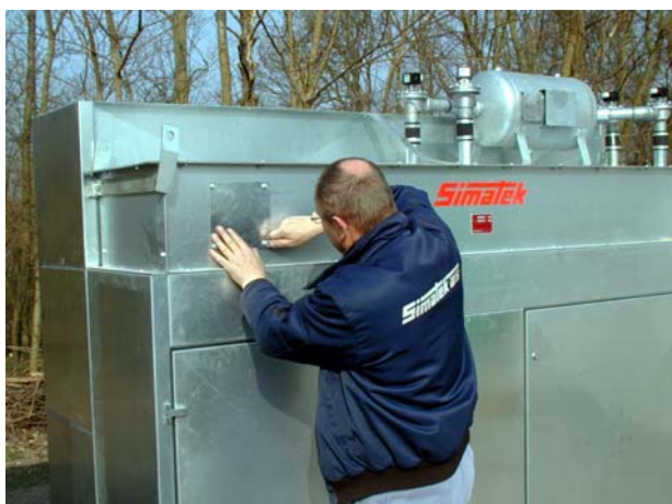
Fig. 1. The cover for the inspection hole is secured with 4 pcs. M8 screws. Loosen the screws with a spanner and remove the cover.
